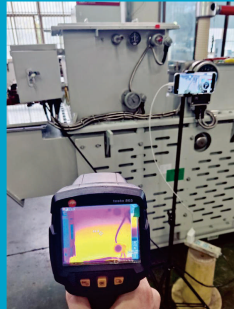
Temperature Rise Test
